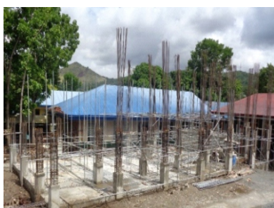
I.T. Laboratory Building
