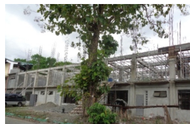
Completion of CAS Building
