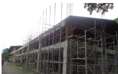
Completion of Gymnatorium
